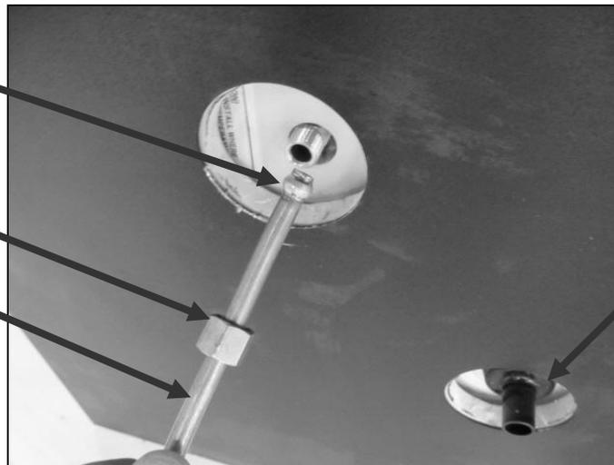
Drain hose connection stub. Slip fit using 1/2"ID flexible drain tubing. Do not use hose clamps as they will damage the coupling.
